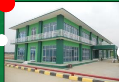
Dry Port 2300 TEUs and Railway Station
