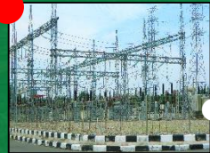
Electricity 150 KV / 60 MVA
