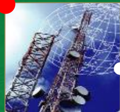
Telecommunication Network & IT (Fiber Optic)
