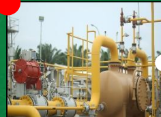
Gas Pipeline 75 MMSCFD
